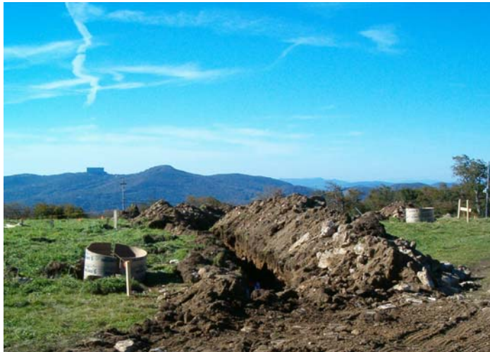
9/23/04 Prep work for tower installation
