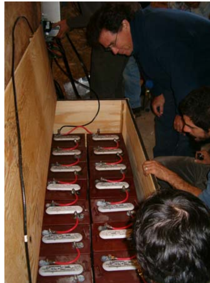
10/21/04 Installing the 48VDC battery bank
