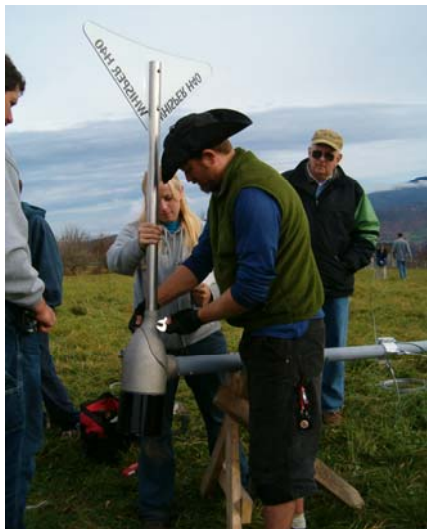
10/19/04 Turbine installation workshop
