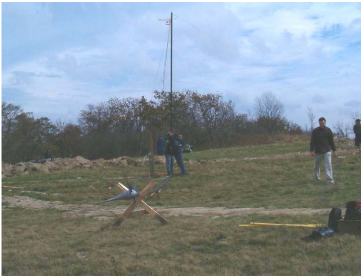
10/18/04 The AirX tower can be raised by human power alone
