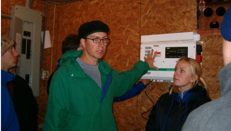
10/18/04 Jay Yeager explaining the Xantrex 4024 inverter
