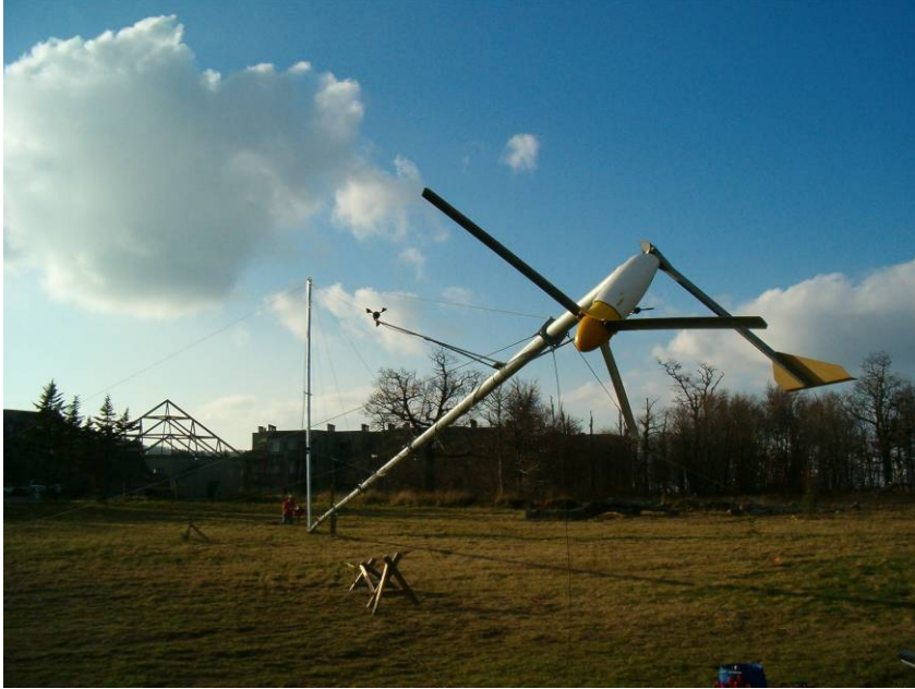
11/1/04 Machine going back up after repairs
