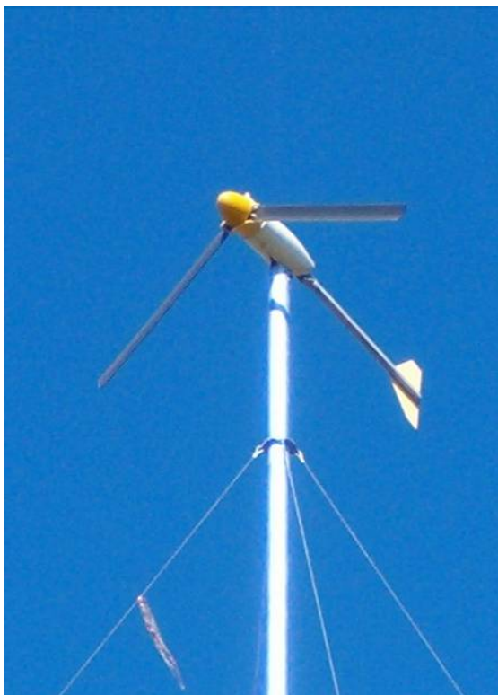
9/22/04 Bergey missing a blade after Ivan
