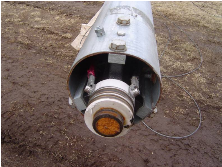
1/12/04 Broken yaw shaft. The landing left a nice dent on the ground.
