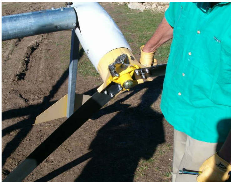
10/4/04 Investigating hurricane damage, broken blade
